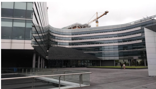
図1 会場全景。Owen G. Glenn Building, The University Auckland。
